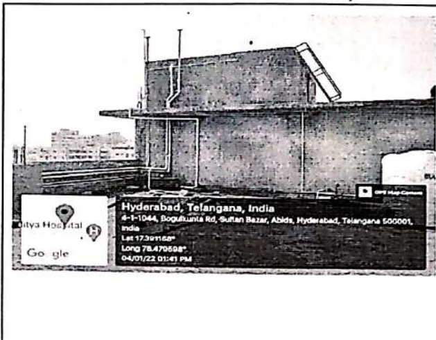
Partition of wastewater( RO Water) and Bore water
