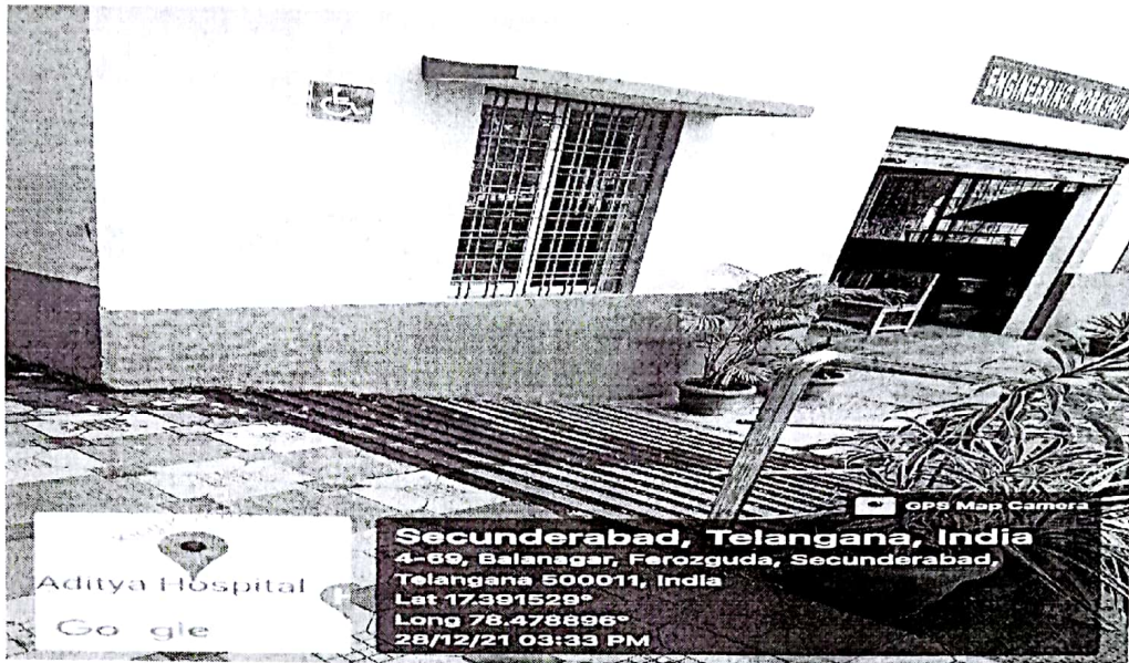
Ramp at 'D' block
