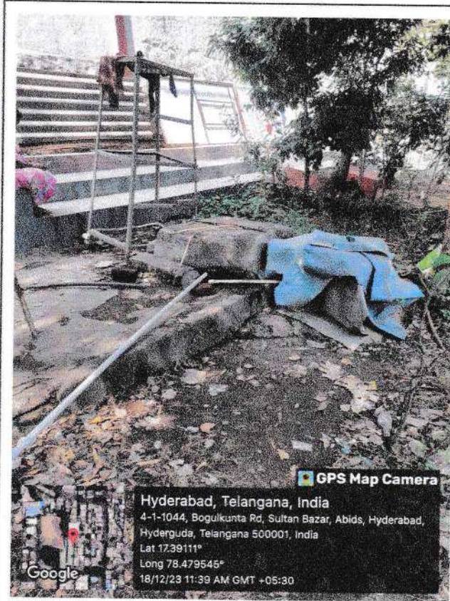
Common dig for water Distribution System
