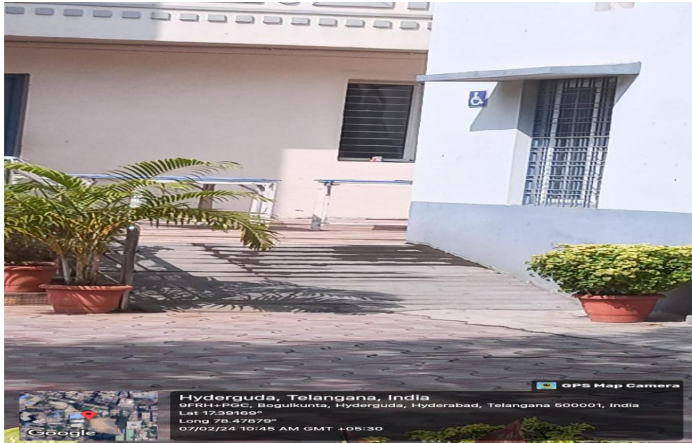
Ramp at 'D' block
