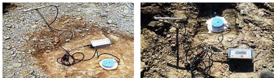
Fig. 4 Ground vibrations monitoring at different locations during blast studies
