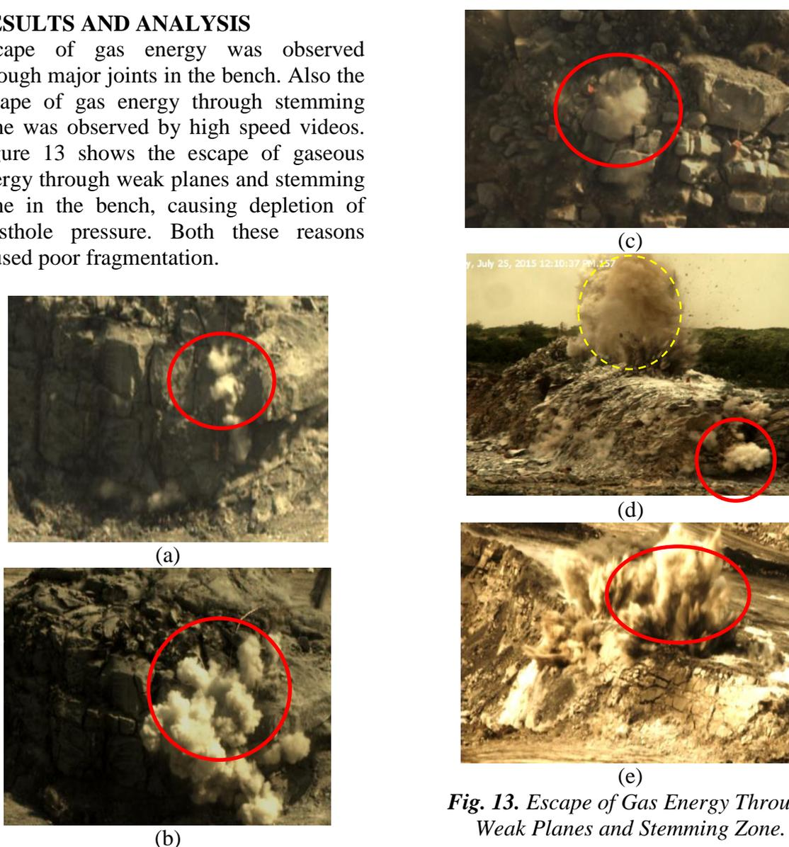
**Fig. 13.** Escape of Gas Energy Through Weak Planes and Stemming Zone.
