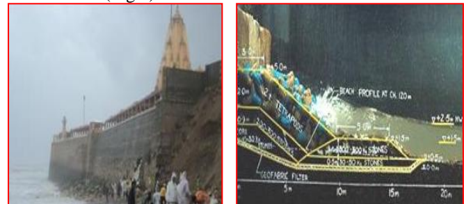
Fig.4 (a): Retaining wall at Somnath temple
