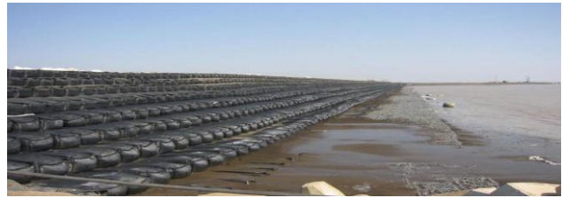
Figure 3. Reclamation bundh using geotextile container
