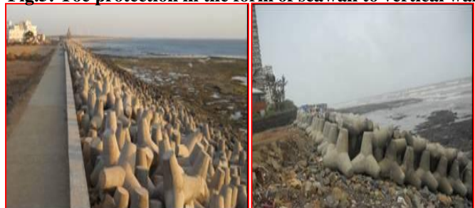
Fig.6: Seawalls with tetrapods in the armour.
