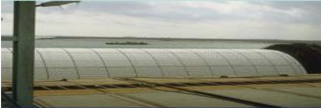
Figure 6. Eastern Scheldt Barrier, The Netherlands
