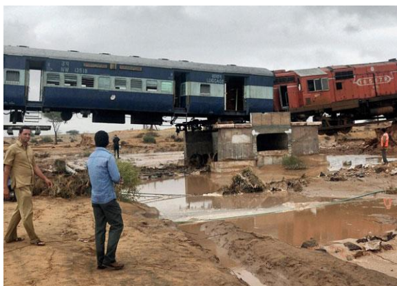
Fig. 1 – Railway Track Washed Away
