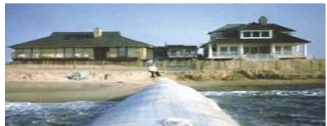
Figure 7. Geotube groyne
