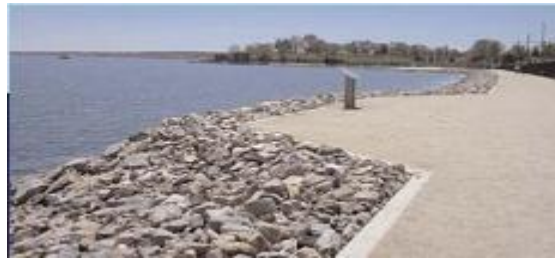
Figure 4. Coastal revetment, CT, USA
