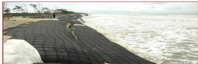
After Installation - During High Tide Figure 2. Installation of geotextile tubes
