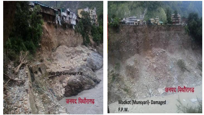
Fig. 9–Damages in Distt. Pithoragarh during flood of June 2013
