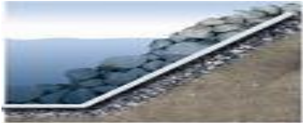
Figure 1. Geotextile preventing coastline erosion
