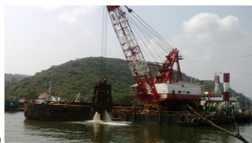
Fig. 7. Blasted Rock Mass Being Dredged. (a) Backhoe Dredger, (b) Grab Dredger.
