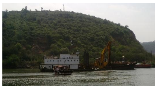
Fig. 7. Blasted Rock Mass Being Dredged. (a) Backhoe Dredger, (b) Grab Dredger.
