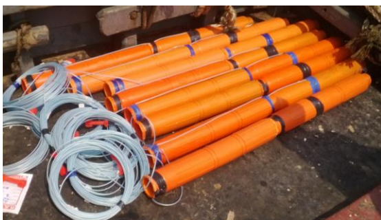
Fig. 6. Explosives in Couplable Tubes and Shock Tube Initiators.
