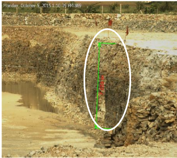
Height of the bench obtained as 7.038m
